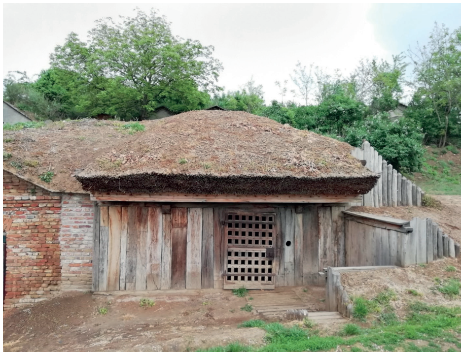
Figure 2 Facade of rebuilt traditional cellar, Sălacea
